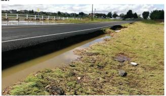
This project has been partially completed - Damage was repaired but the lack of adequate box culverts to handle the 100-year flood will result in future damage. The Town of Frederick Stormwater Master Plan will identify this project as a priority.
