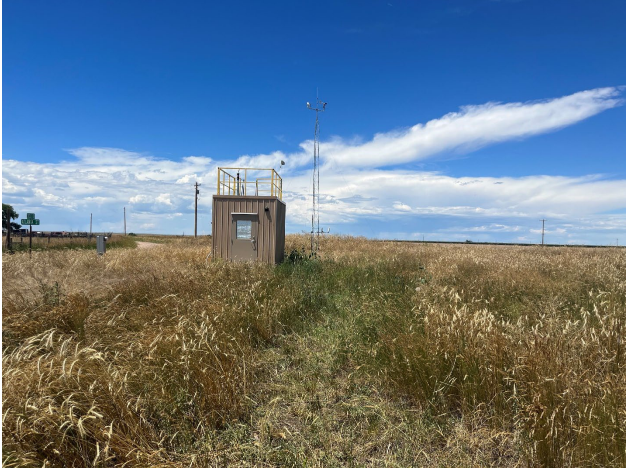
Figure 25: Photo#12: Looking West.
