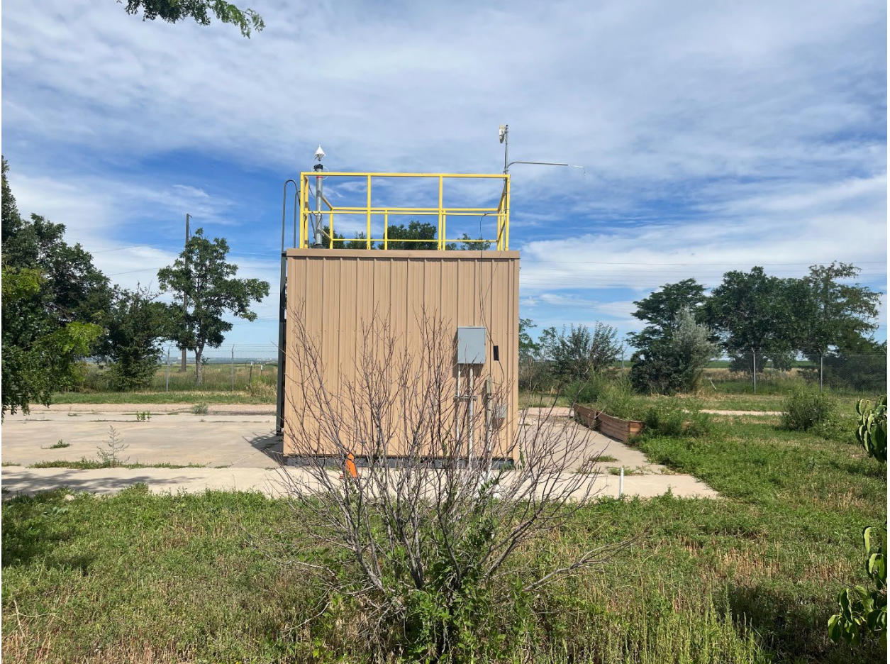
Figure 10: Photo#3: Looking East
