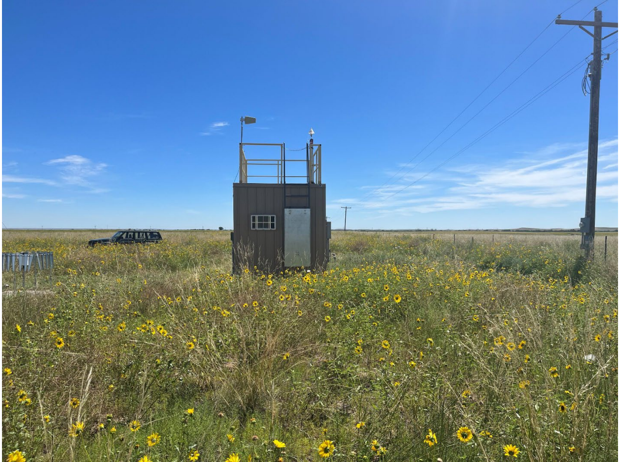
Figure 17: Photo#7: Looking East
