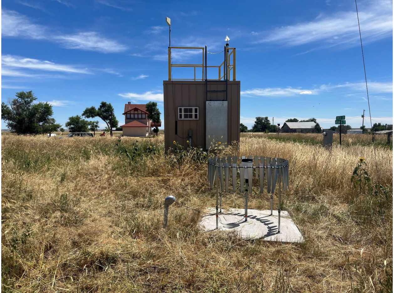
Figure 24: Photo#11: Looking East.
