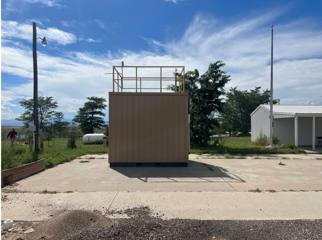
Figure 11: Photo#4: Looking West
